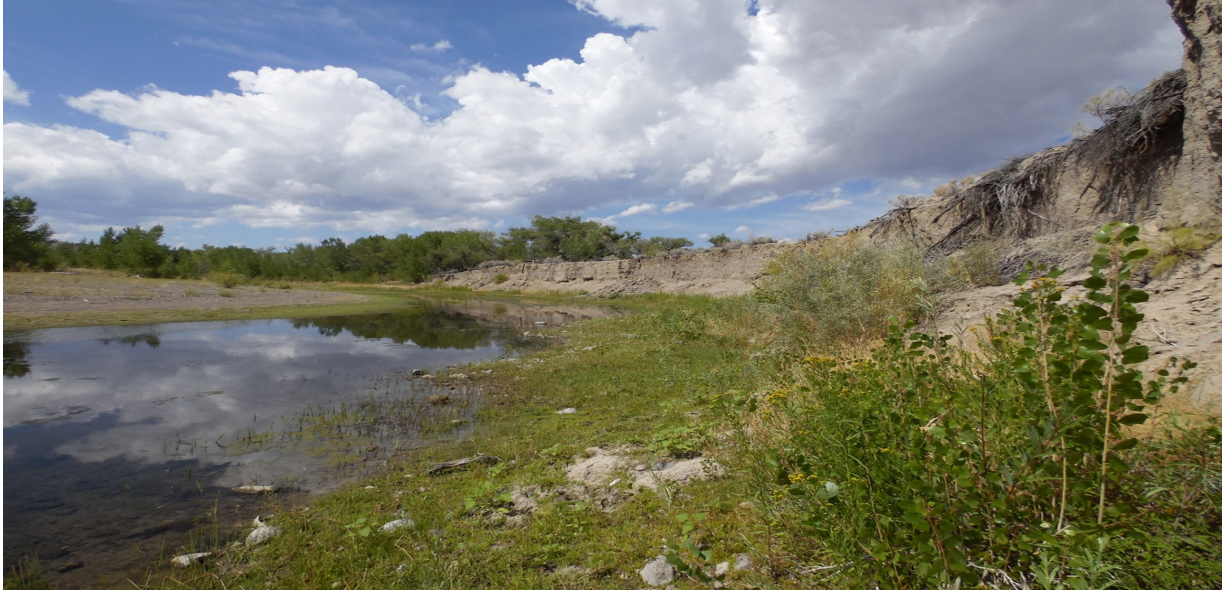
MCR 049 and visible bank erosion
