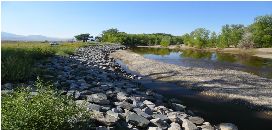
MCR 048 Emergency Repair Work
